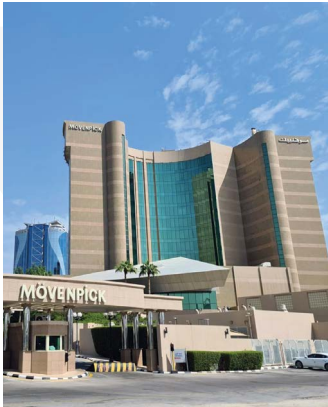
Movenpick Hotel Al Khobar - KSA
