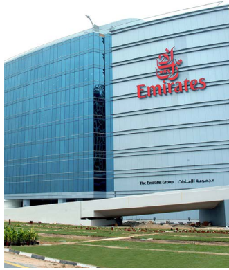
Emirates Airlines Headquarters - Dubai
