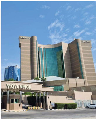
Movenpick Hotel Al Khobar - KSA
