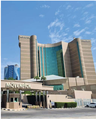
Movenpick Hotel Al Khobar - KSA
