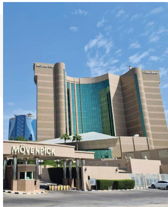
Movenpick Hotel Al Khobar - KSA
