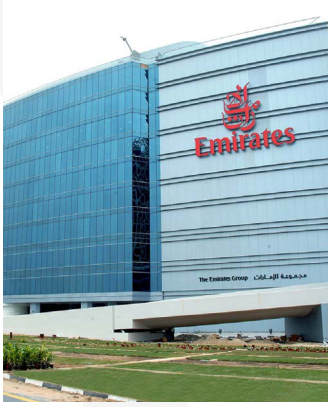
Emirates Airlines Headquarters - Dubai
